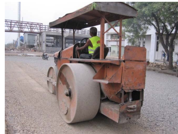
Compaction by a 10 tonne roller
