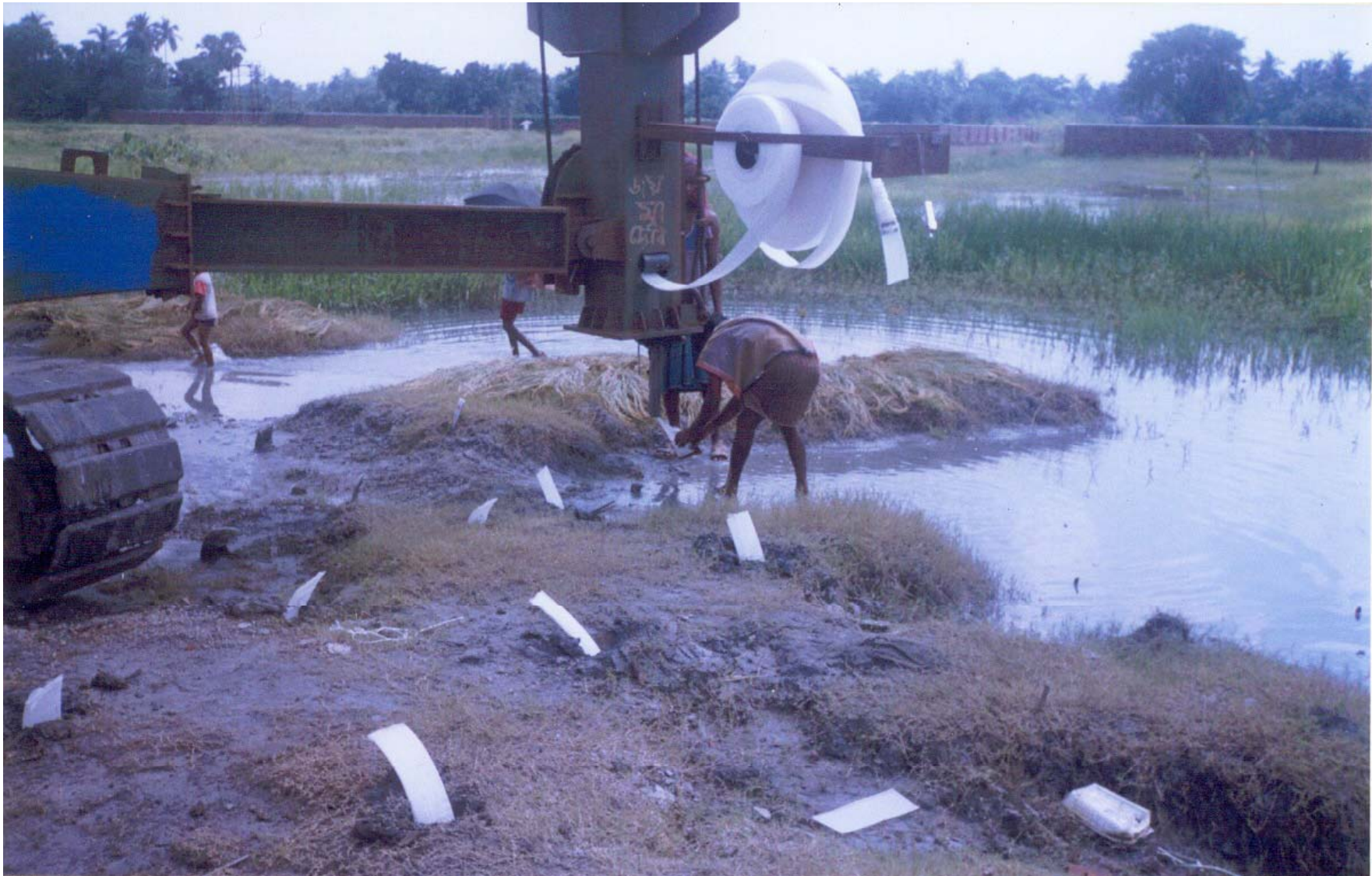
PVD being pushed into the ground
