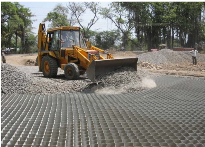
Stone aggregate filled in geocell pockets
