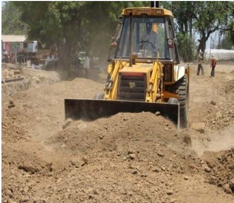
Preparation of ground
