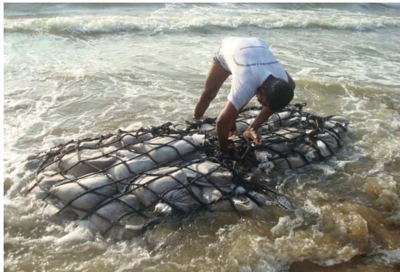
TYING OF ROPE GABIONS
