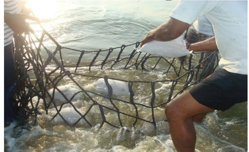
PLACEMENT OF GEOBAGS
