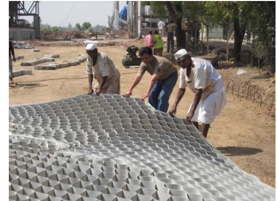
Stretching of the geocell layer
