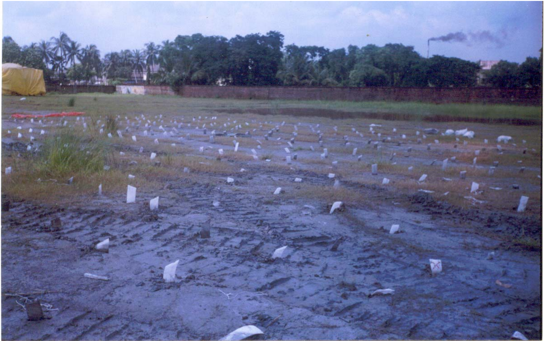
General view after installation of PVD's at a site
