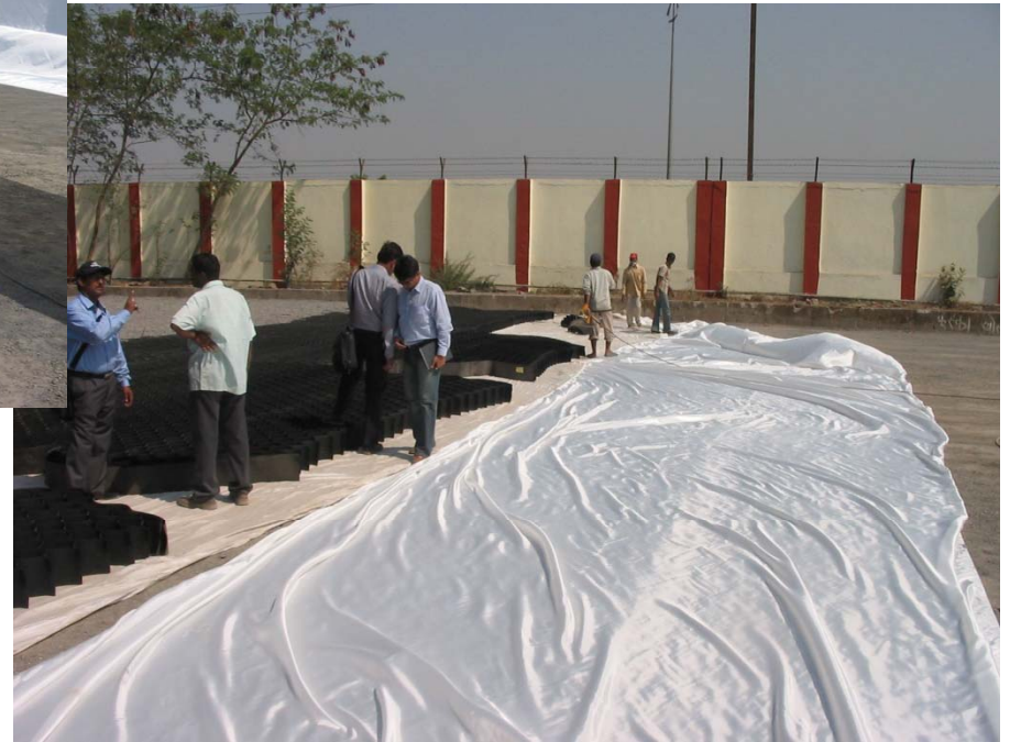
Geotextile separator being laid on the ground surface at a container yard
