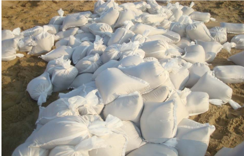
SAND FILLED GEOBAGS
