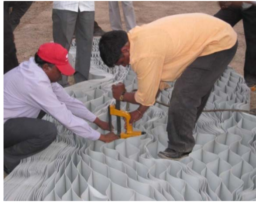
Stapling to join different geocells
